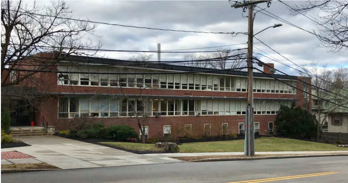
Figure 2: Academic Center view from Fisher Ave.
