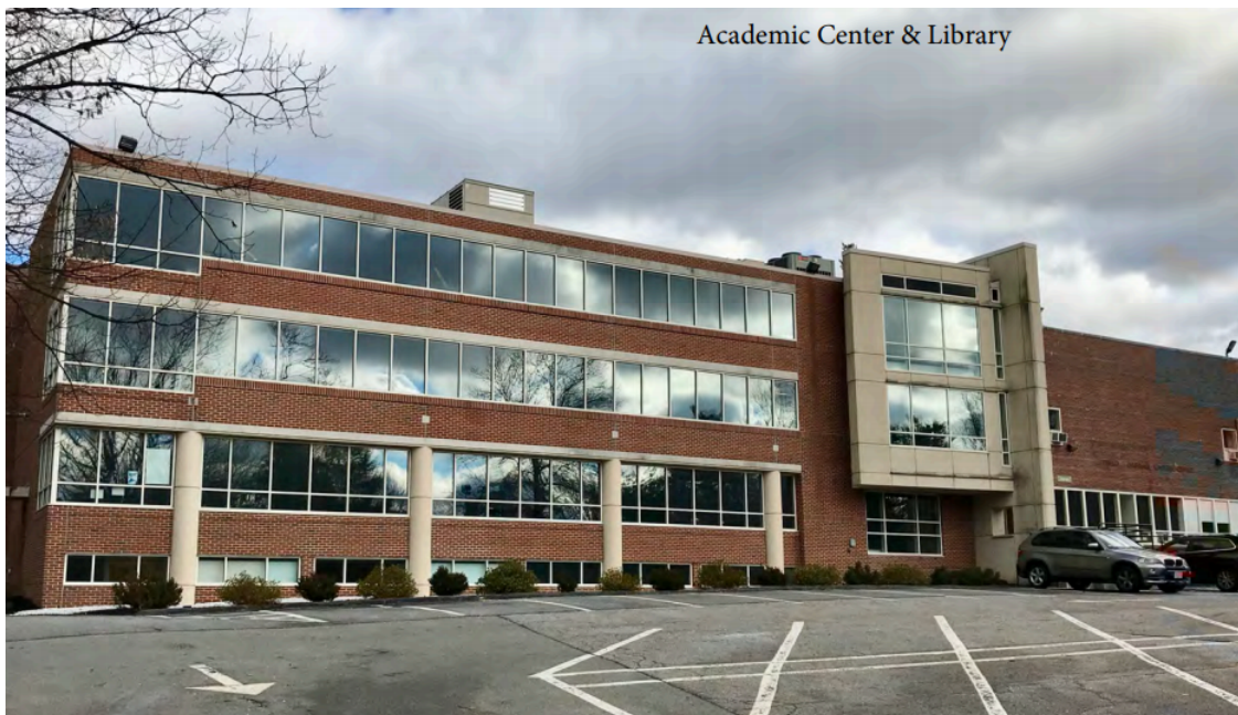
Figure 3: Rear of Academic Center showing 1997 Library addition
