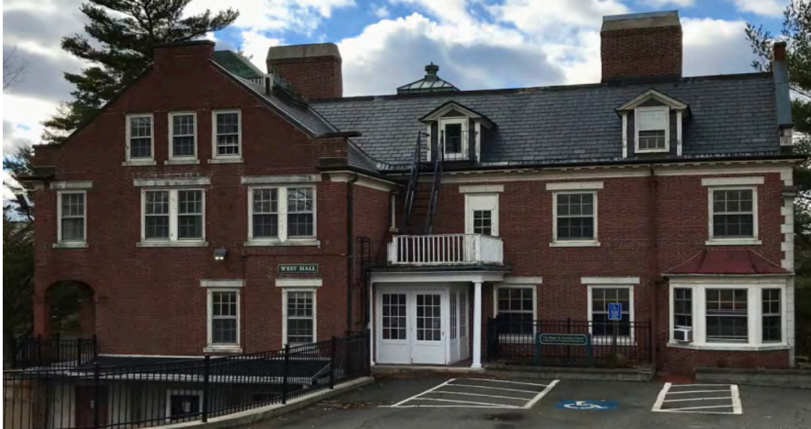
Figure 3: Rear View of West Hall
